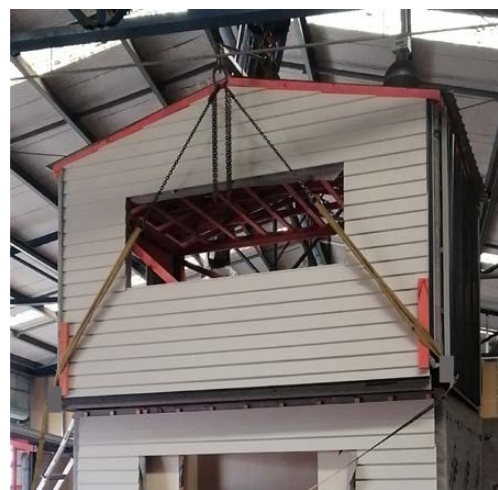
Modules being lifted in the factory
